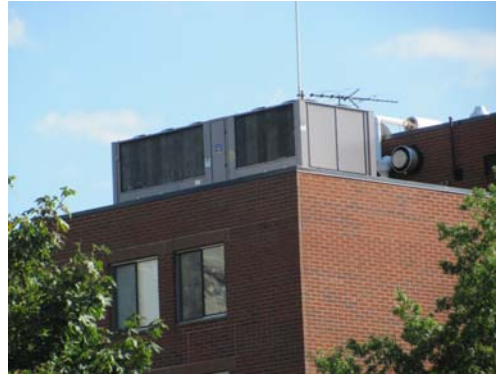
pre retrofit work on roof HVAC system
